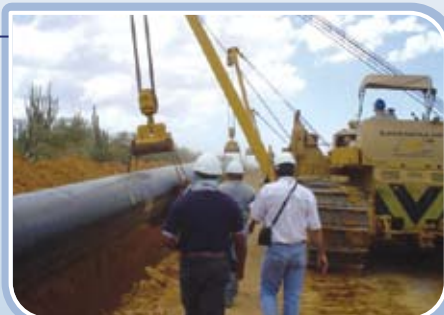
Laying the pipeline
